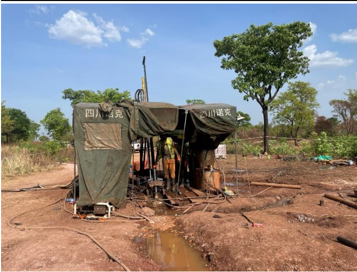
Figure 14: Compact diamond drill rig at BDT1
